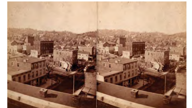
VIEW FROM TYMAN'S BUILDING, STAPLETON
